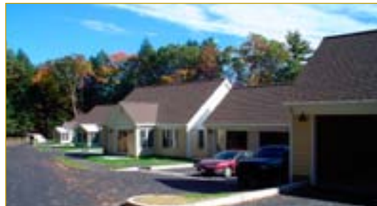
ROCKRIDGE COTTAGE EXPANSION Northampton, Massachusetts 7 Independent Living Cottages
